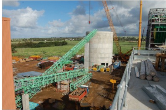
Conveyor Construction
