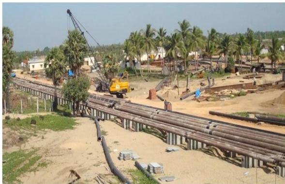
Laying of Jacketed Piping at Cudallore
