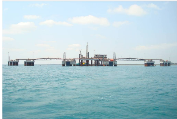
Cat walk structures & piping for VCM line
